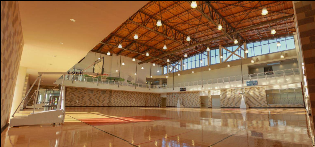
Interior View 2 Court Gymnasium
